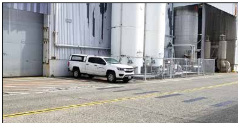
BEFORE: Old dark painted crosswalk led to vehicular roll-up door. Pedestrians then had to cross in front of the door creating a hazard.
