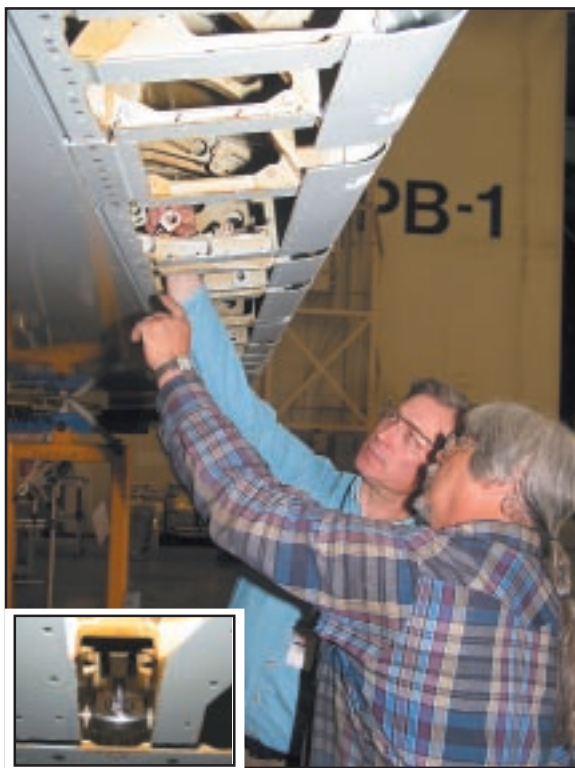
Lyn Hallenius (foreground) shows Business Rep Zack Zaratkiewicz how installing the clevises after the sealing process is complete will save about 4 hours per wing. Photo inset: Shows the clevises on the wing.
