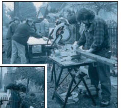
Above: Duane Roope cuts wood for the railing of a ramp in Seattle.
