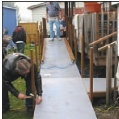
Members attach the painted plywood to the recent Federal Way ramp.
