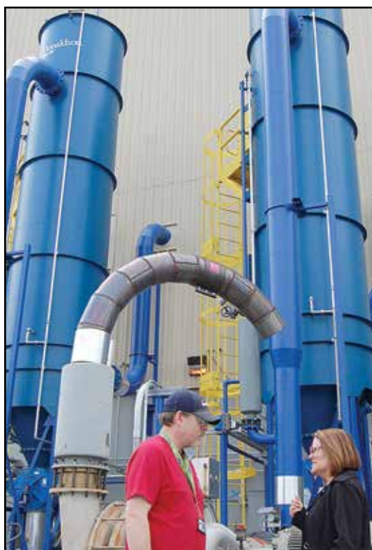
Patrick Tingley and Business Rep Grace Holland discuss the new vacuum system that makes it safer for the operators to do their job and also cuts hours off their work process.
