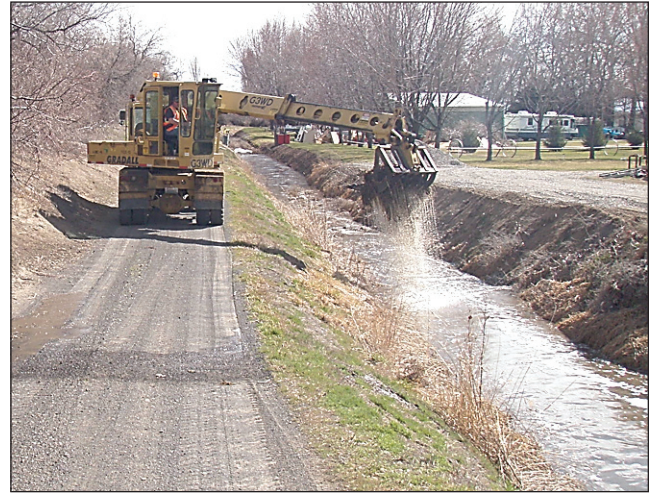
Workers clear debris from an irrigation ditch to prevent flooding.
