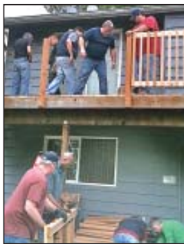
Above: Rebuilding the railing system for a home in Bothell.
