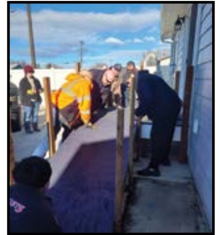
The finishing touches before it receives the final check.
