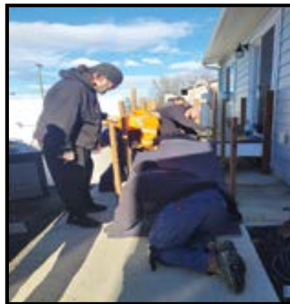
The second part of the ramp comes to life.
