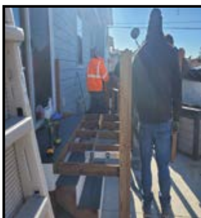
The start of the build - framing the ramp.
